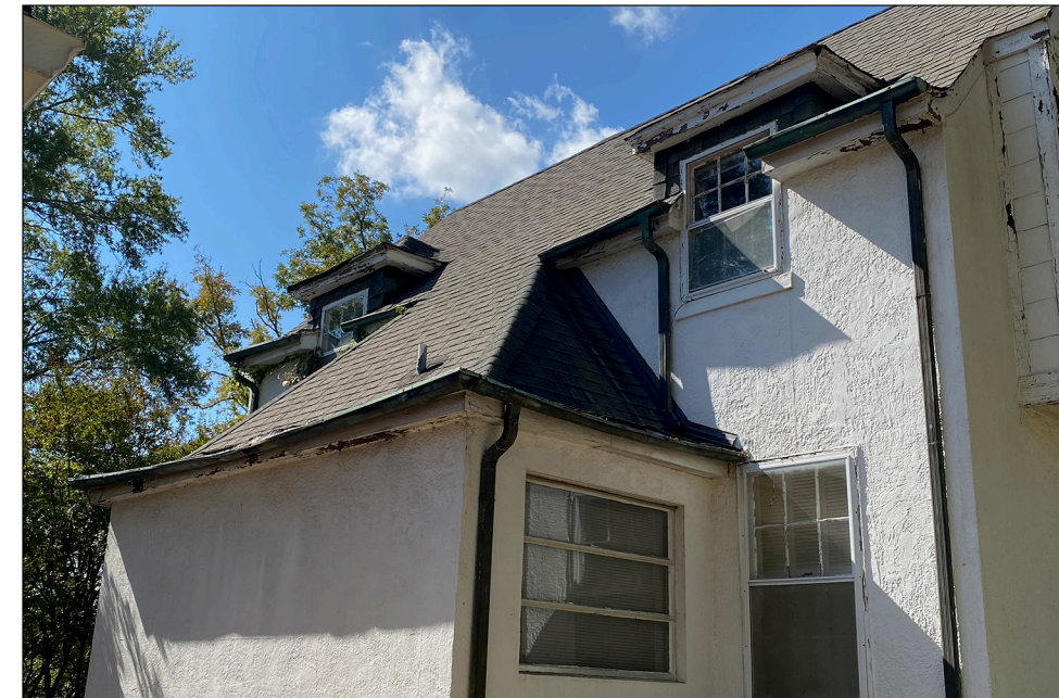
right diagonal view
