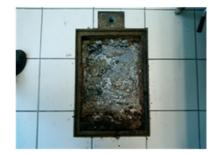
Figure 69: Grease trap overflow is a hazard to kitchen employees.
