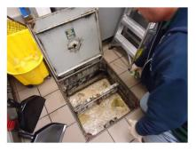
Figure 36: Grease trap installed flush with the floor (an in-floor trap).
