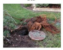
Figure 60: Roots removed from the grease interceptor (root intrusion can completely clog the interceptor).
