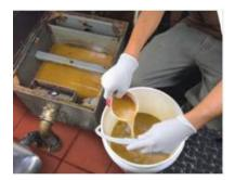
Figure 38: Removing grease from the grease trap.
