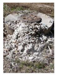
Figure 68: Grease interceptor overflow.
