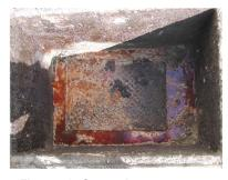
Figure 58: Grease interceptor not working.
