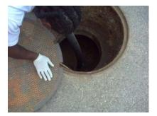
Figure 47: Vacuuming out the contents of the interceptor.
