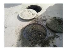
Figure 67: Grease interceptor completely full. Heavy lids can be lifted up under pressure and grease start overflowing.
