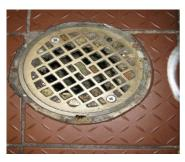
Figure 55: Debris in the floor drain (floor was not swept before mopping).
