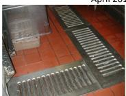
Figure 27: Floor drain screen.
