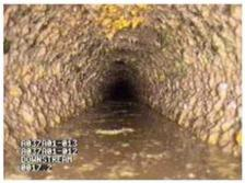
Grease in the pipe. It generally accumulates from the top of the pipe down while other debris accumulates from the bottom up.
