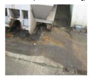
Figure 57: Waste leaks in the garbage and grease recycle storage
