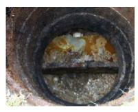
Figure 59: Too short outlet tee allows short-circuiting.
