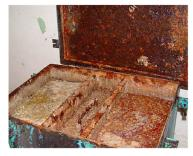
Figure 61: Severely corroded metal grease trap (these traps are highly prone to corrosion).
