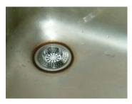
Figure 26: Sink drain screen.
