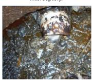
Figure 63: Missing inlet tee allows FOG buildup in front of discharge pipe.
