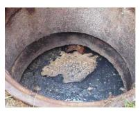
Figure 64: Missing outlet tee allows floating FOG to escape into the sewer system.
