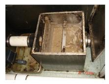
Figure 35: Grease trap installed above ground.
