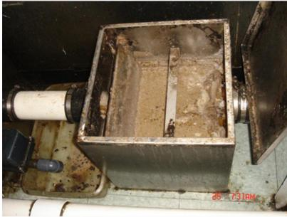
**Figure 35: Grease trap installed above ground.**
