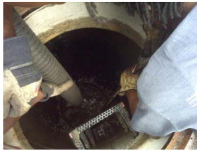
**Figure 48: Use of high pressure water and suction hose.**
