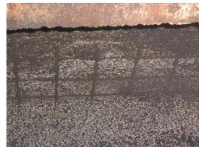
Figure 62: Exposed re-bar in a corroded concrete interceptor.
