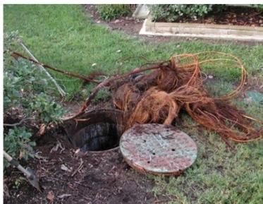
Figure 60: Roots removed from the grease interceptor (root intrusion can completely clog the interceptor).
