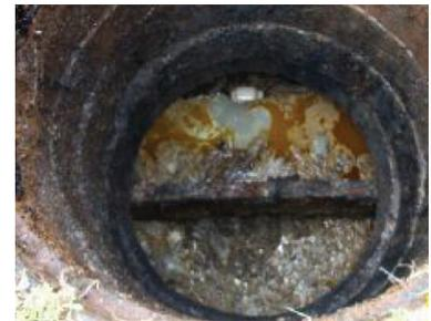
Figure 59: Too short outlet tee allows short-circuiting.
