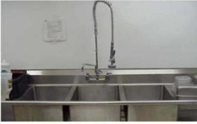
**Figure 25: Three-sink dishwashing system.**
