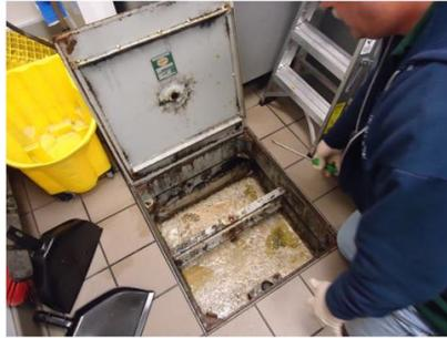
**Figure 36: Grease trap installed flush with the floor (an in-floor trap).**
