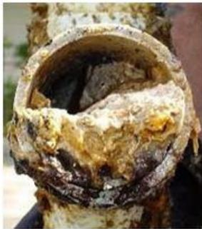
**Figure 1: FOG deposit clogging the sewer pipe.**
