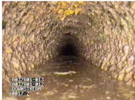
**Figure 2: FOG accumulated on the wall of sewer pipe.**
