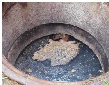
Figure 64: Missing outlet tee allows floating FOG to escape into the sewer system.
