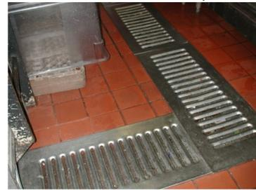
**Figure 27: Floor drain screen.**
