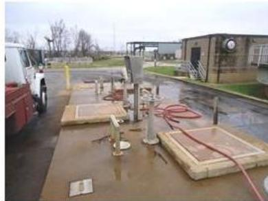
**Figure 53:** Three subsurface holding basins for questionable or more toxic hauler loads.
