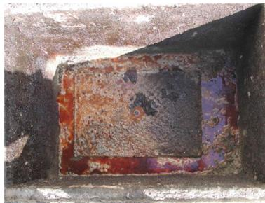
Figure 58: Grease interceptor not working.
