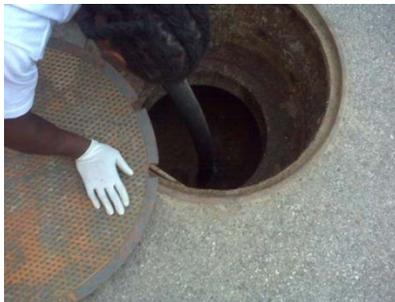
**Figure 47: Vacuuming out the contents of the interceptor.**
