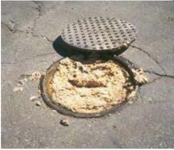
**Figure 41: Interceptor filled with grease to the top.**
