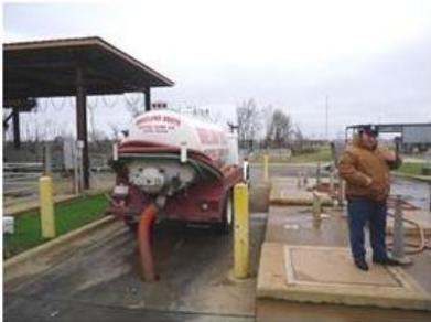
**Figure 52:** A hauler truck discharging into a receiving hole in a receiving area adjacent to the plant's influent pump station.
