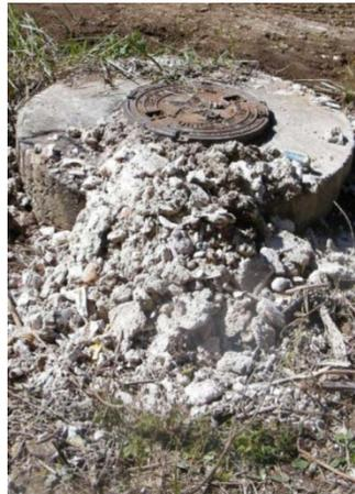
**Figure 68: Grease interceptor overflow.**
