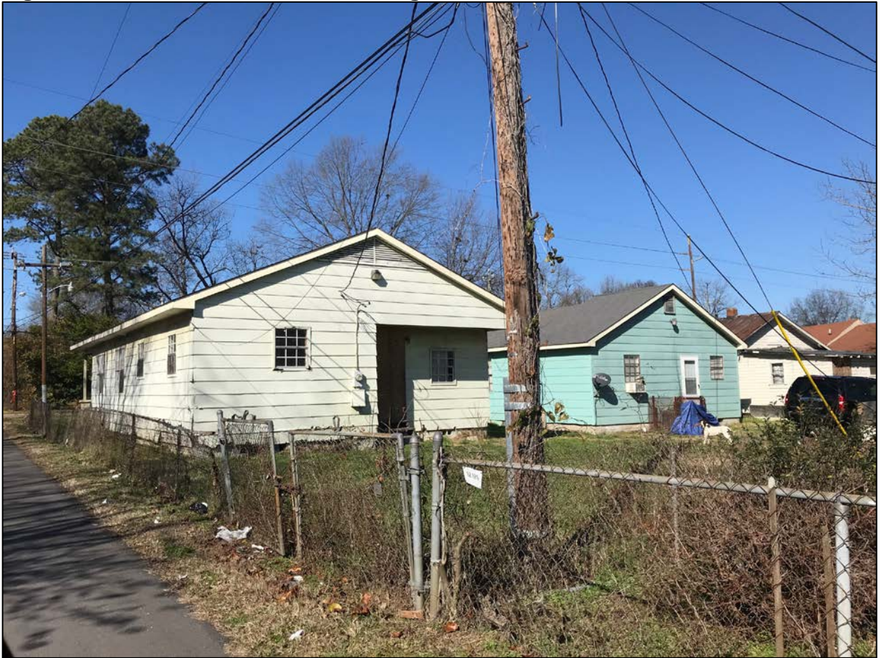
Figure 22. Overhead Powerlines in Neighborhood
