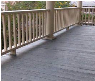
Porches and railing
