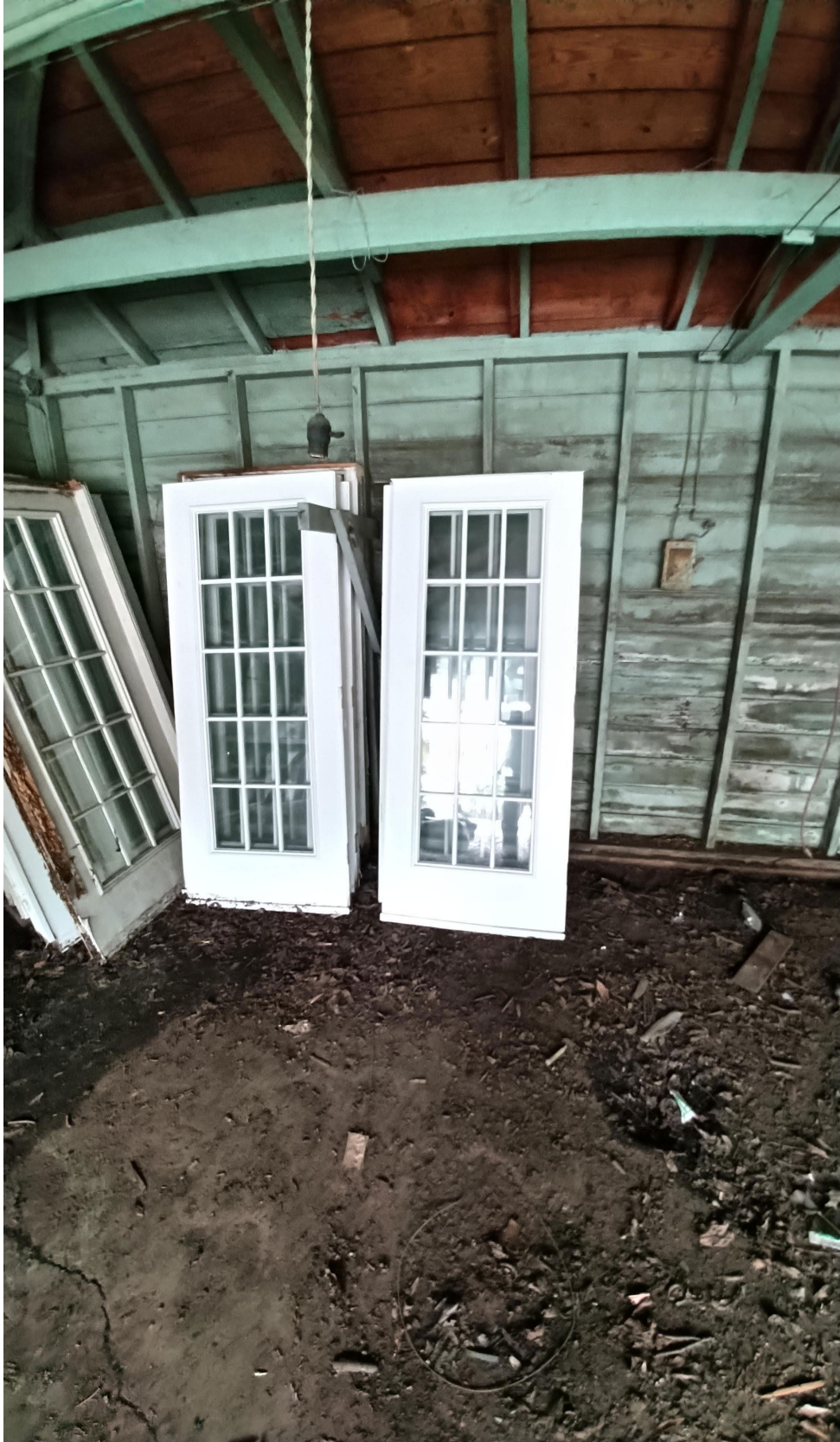
Old windows: 15-lite fixed metal clad
